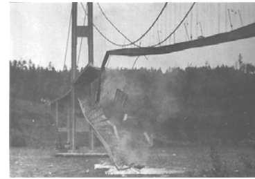
Tacoma Narrows Bridge (wind-induced roadway oscillation)
