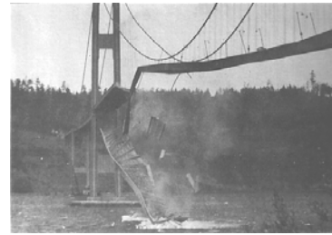
Tacoma Narrows Bridge (wind-induced roadway oscillation)
