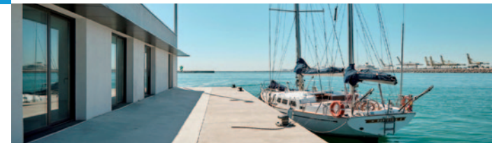
The Barcelona School of Nautical Studies (FNB) has new facilities in the Espai Vela, in the Port of Barcelona, with mooring points, space for up to seven boats and a davit for raising and lowering the boats.
