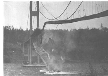
Tacoma Narrows Bridge (wind-induced roadway oscillation)
